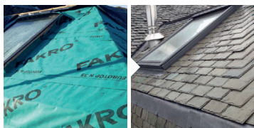
SLATE ROOF Before/After
