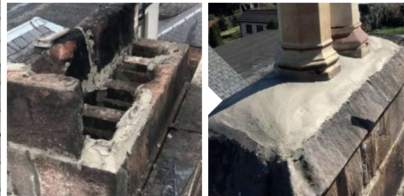
CHIMNEY RESTORATIONS Before/After
